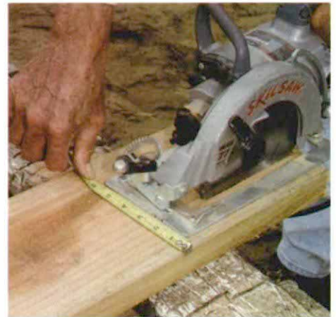
Saw base can help gauge ripping widths. Knowing the distance between the blade and the edge of the saw base lets you rip many widths without a line. Here, the author has estimated ½ in. beside the base for a 2-in. rip.
