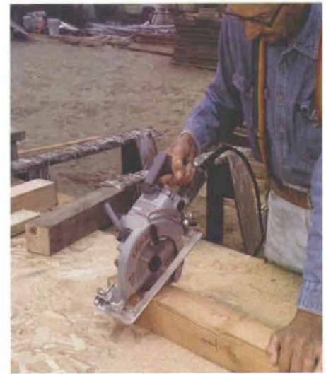
Perfect post cuts in a snap. Cut side one as you would a 2x4 (top). Next, rotate the 4x on edge and cut side two (center). Keeping the blade in the kerf, roll the 4x forward and plunge through side three in chopsaw fashion (bottom). The saw kerf from the first square cut aligns the next two.
